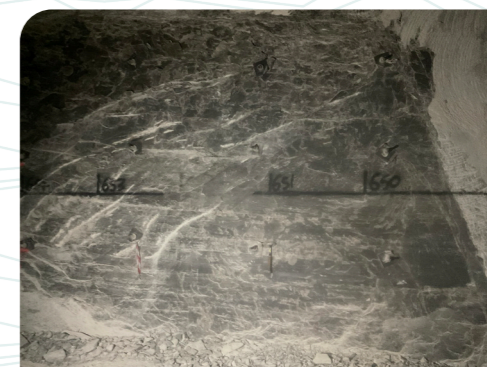
Side wall through the polyhalite – bedding clearest at base along with rock bolts and survey markers. White marks are machine scratches. Geological hammer for scale.
